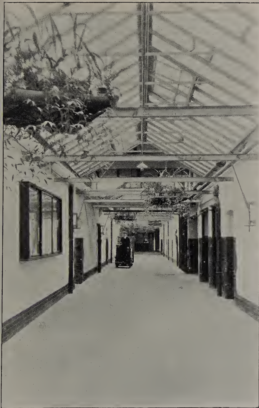
A TYPICAL CORRIDOR SHOWING HANGING PLANTS
